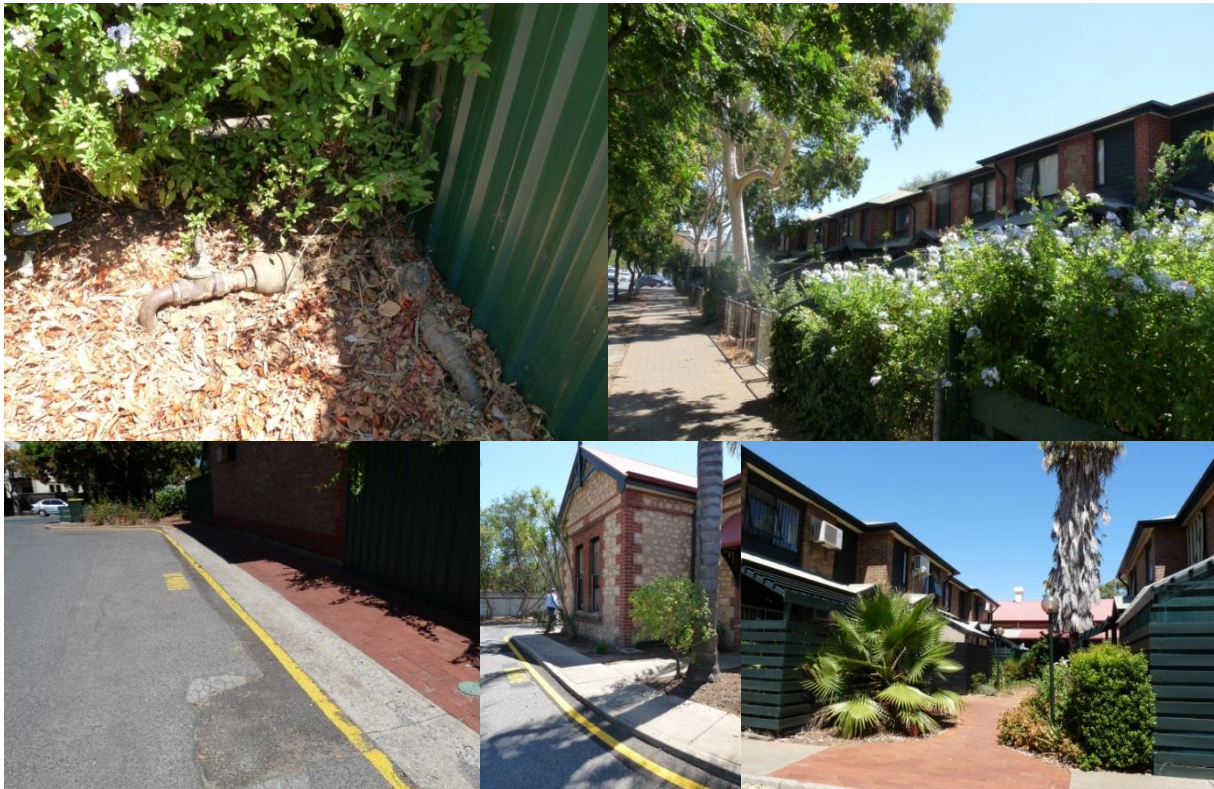
Clockwise from top left: Original SA Water meter feeding site; front block of attached townhouses fed by original SA Water meter; back block of townhouses; new internal pipework required to isolate into two groups; new SA Water meter added and internal pipework extensions to feed the back blocks of townhouses.
