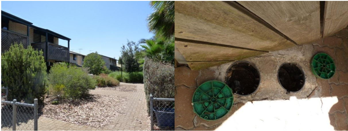
Pictures left to right: Townhouses, flats and common gardens at site 4; two private flow meters - one servicing upstairs flat, one servicing downstairs flat.
